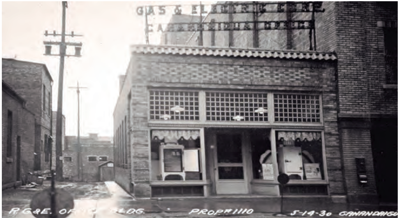
Photo of the first Rochester Gas and Electric (RG&E) building, 1930. Avangrid Service Company.
